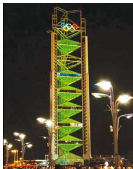
The Ling Long Tower was used to stream international broadcasts from the Olympic village during the games. This 132 m high LED-lit tower features seven pyramid structures.
