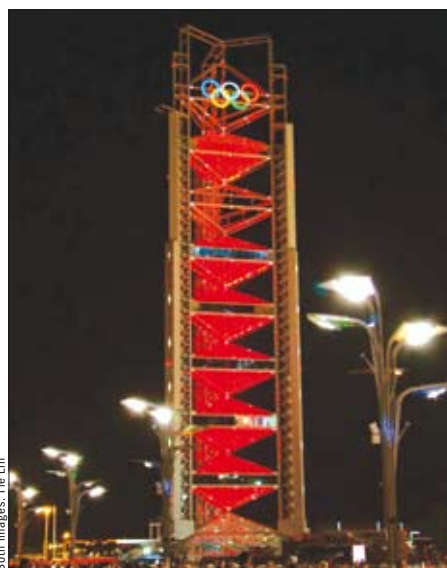
The Ling Long Tower was used to stream international broadcasts from the Olympic village during the games. This 132 m high LED-lit tower features seven pyramid structures.
